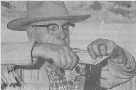
STEP 5 – Trim away excess patching material with a sharp knife.
