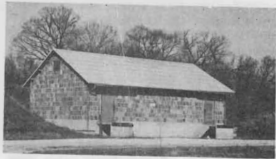
FIGURE 21 — Finished powder is placed in large cans and stored in magazines such as this prior to canistering for distribution. For safety, magazine buildings are situated a distance from each other.
