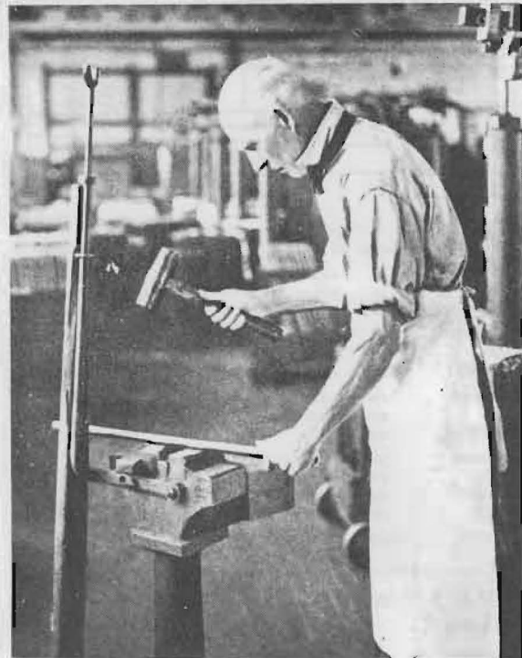
FIGURE 7 — In the days of yore, crooked barrels were straightened by pounding the barrel against lead blocks with a lead hammer.
